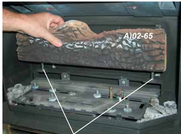
Pins on Rear Log Support
